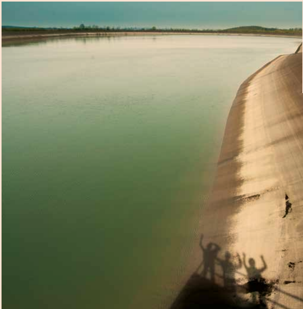
Top: Erzhausen pumped-storage hydropower plant in Germany
